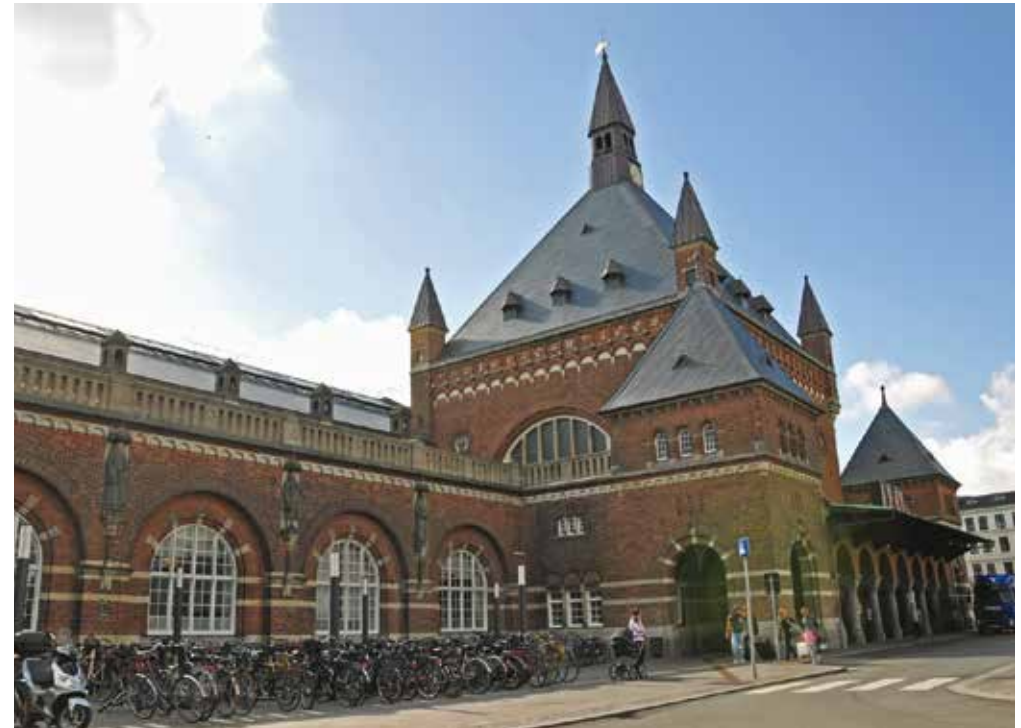
Main entrance of Copenhagen station. Source: UIC
