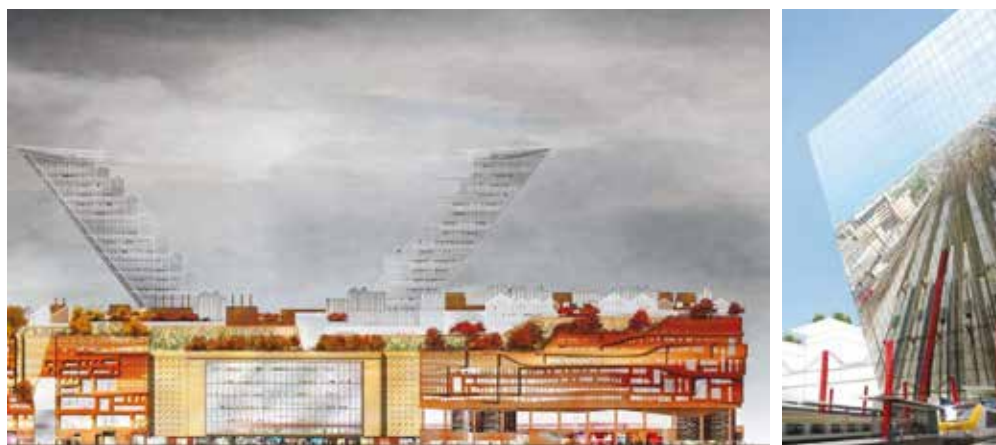
A modern, 550m-long façade and a transparent V-shaped building.
