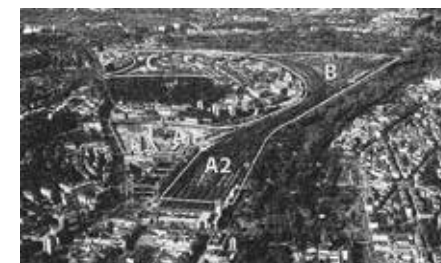
Stuttgart 21 project: La vie du rail. October 2010 - UIC 2013.
