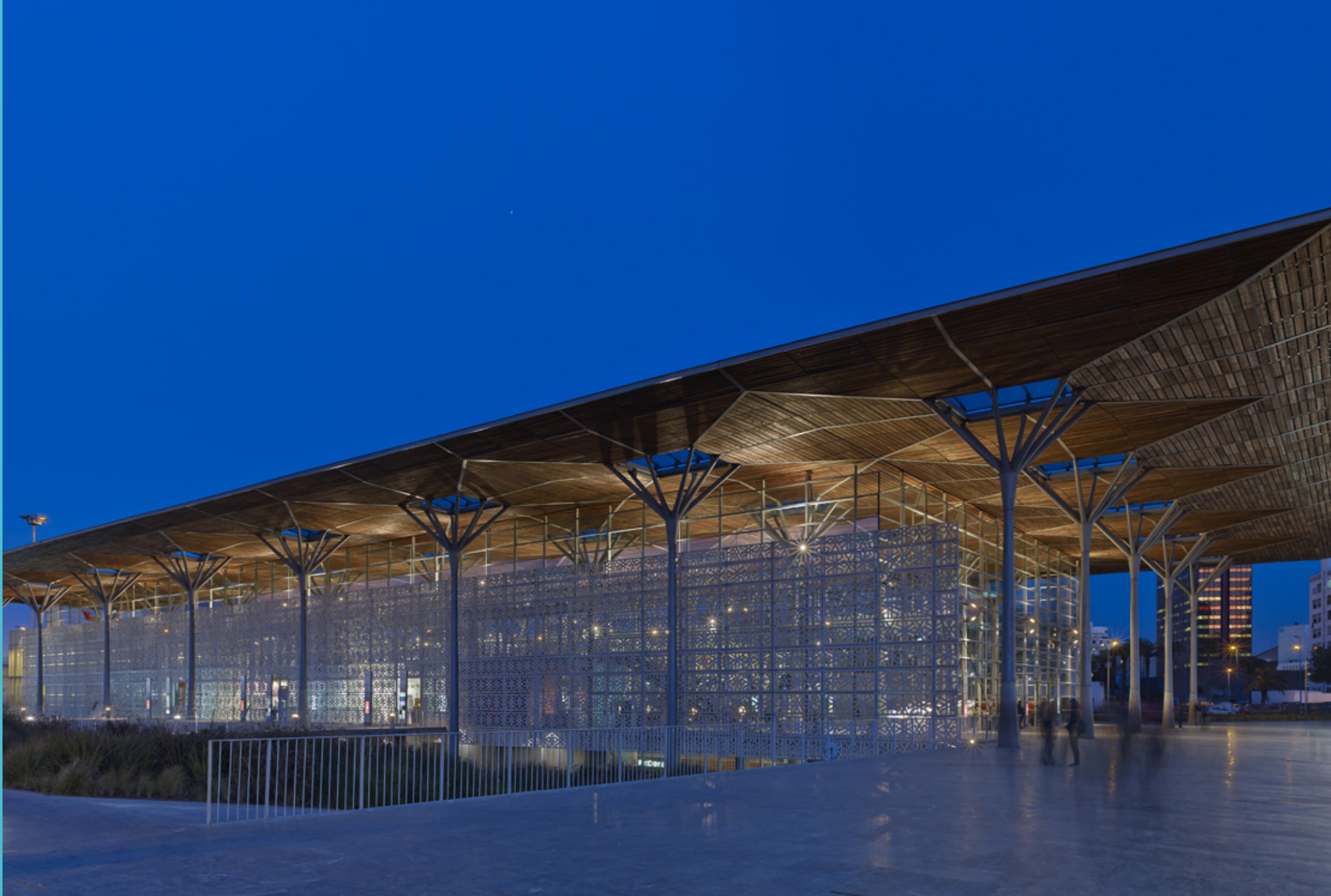
The new Casa-Port Station, Casablanca, Morocco. February 2015. AREP/ Photographer: Didier BOY DE LA TOUR.
