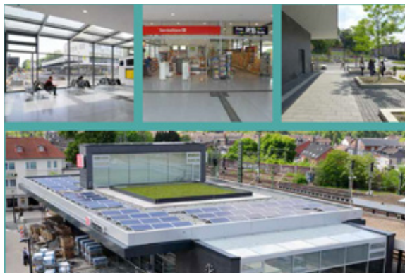
In Horrem in Germany, Deutsche Bahn has developed an innovative concept of passenger building combining up-to-date ecological standards with a high level of customer comfort. Above is the "StationGreen building" with its living or green roof and photovoltaic panels. (Source: Brunel Awards 2014)
