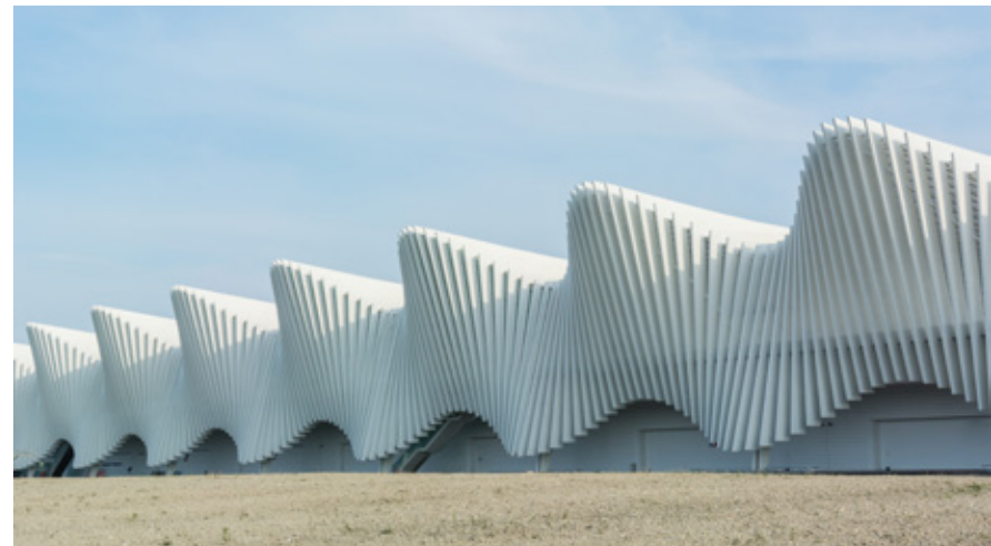
Reggio Emilia Station, a project designed by the architect Santiago Calatrava, was opened on June 8th 2013. Its sinusoid or wave form is created by a succession of porticos with closed sections and differing geometrical shapes. (Source: Fotolia)
