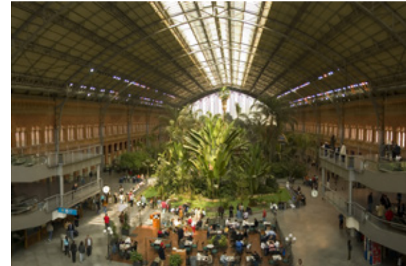
Atocha Station, Madrid (Spain). A green space has been created within the station so travellers can appreciate the local flora and fauna as soon as they step off the train. (Photo courtesy of Rafael Ramirez Lee)
