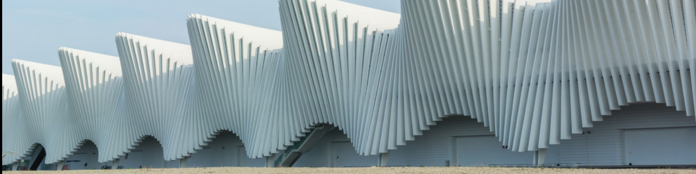
Reggio Emilia Station, a project designed by the architect Santiago Calatrava, was opened on June 8th 2013. Its sinusoid or wave form is created by a succession of porticos with closed sections and differing geometrical shapes. (Source: Fotolia)
