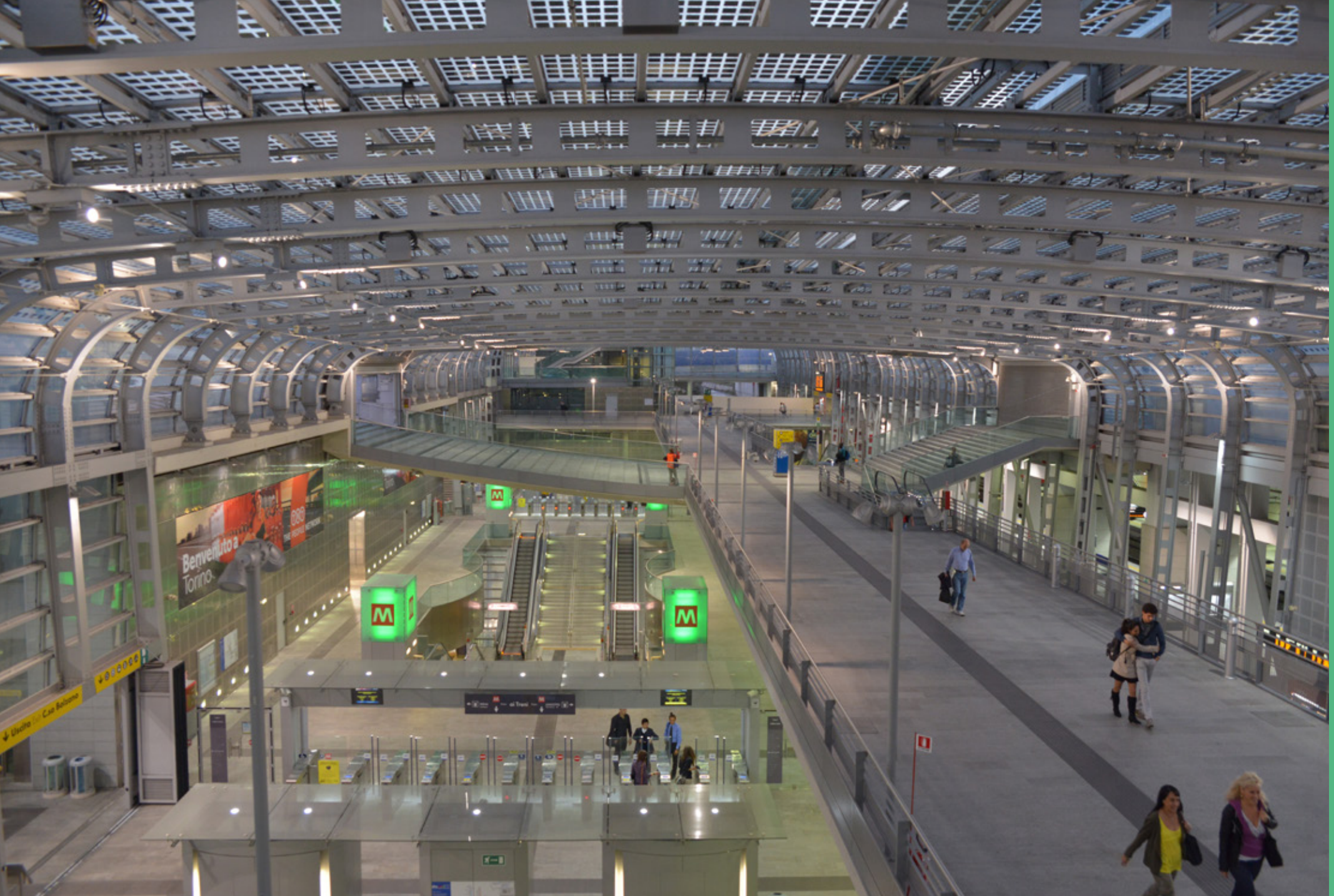
New RFI Turin Porta Susa Station, Italy: view of the concourse from above. October 2014. AREP/ Photographer: Mathieu Lee Vigneau. Architects: Jean-Marie Duthilleul and Etienne Tricaud, Silvio d'Ascia in association with A .Magnaghi.
