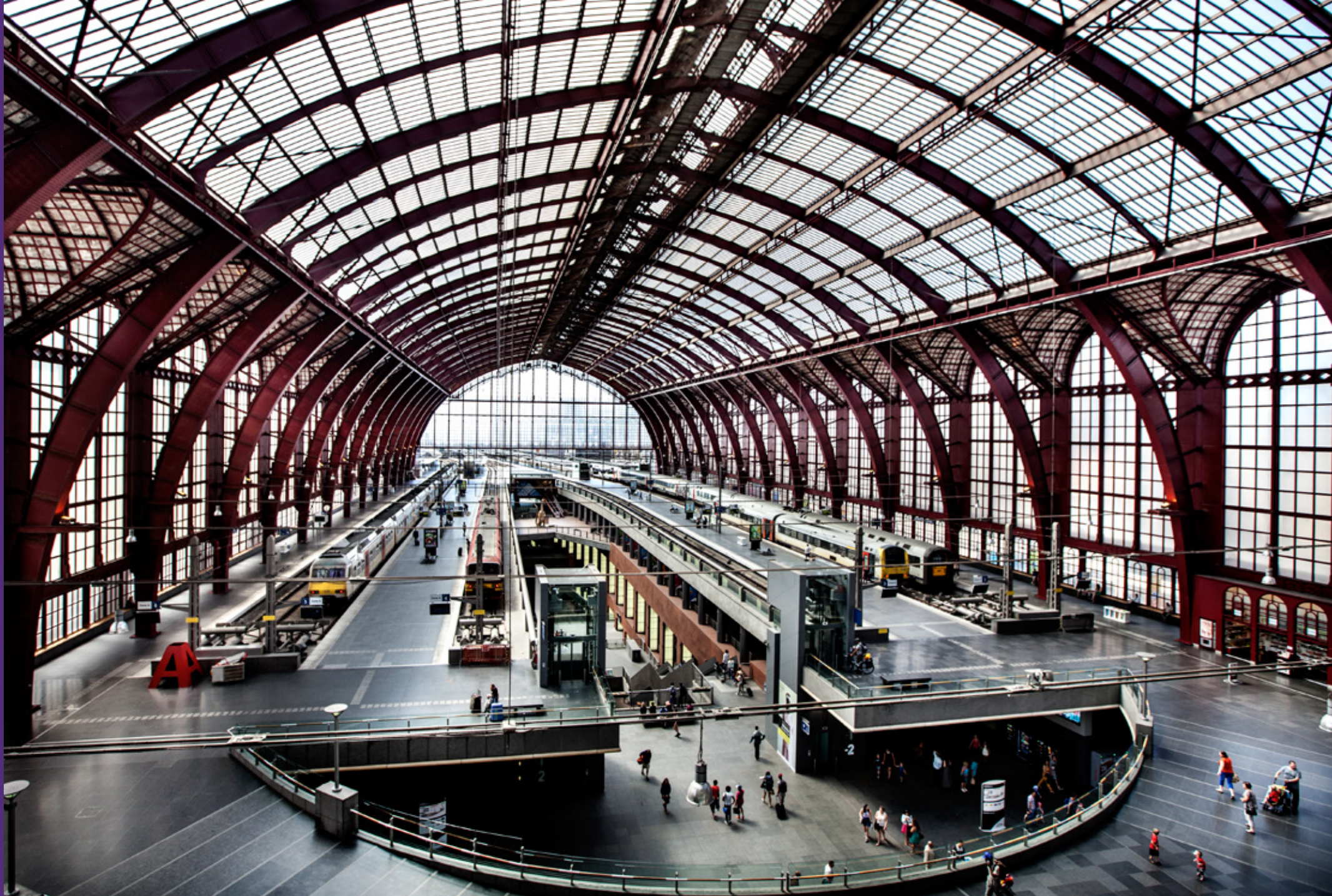
Antwerp Station, Belgium. (Source: SNCB)
