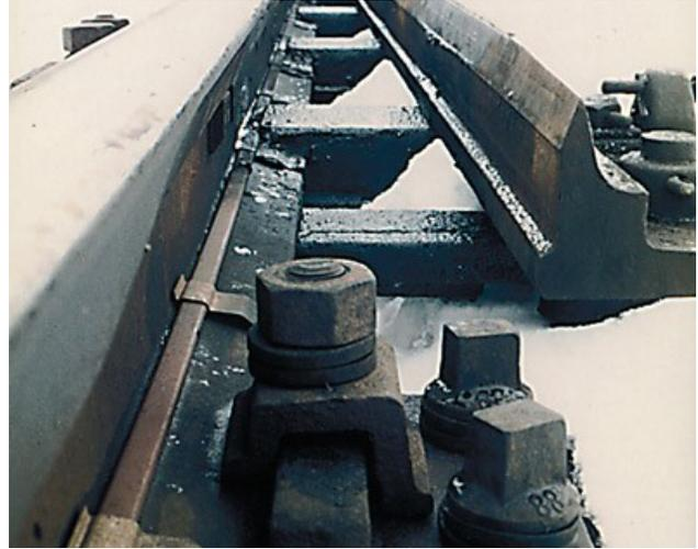
Figure 2: Railway switch equipped with electrical heater. Source: railway-technology.com.
