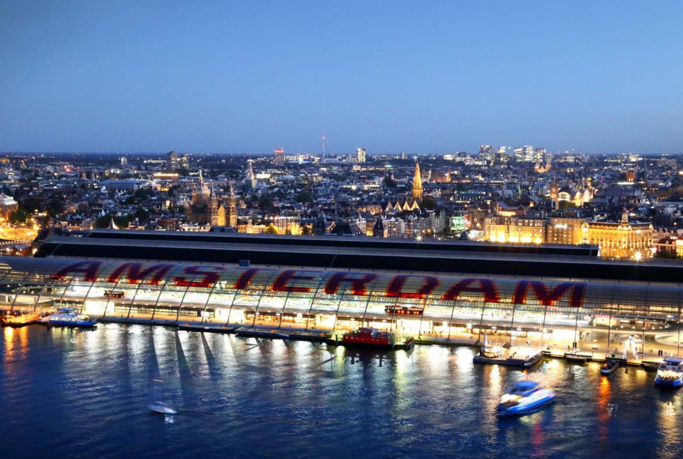
Amsterdam railway station, the Netherlands
