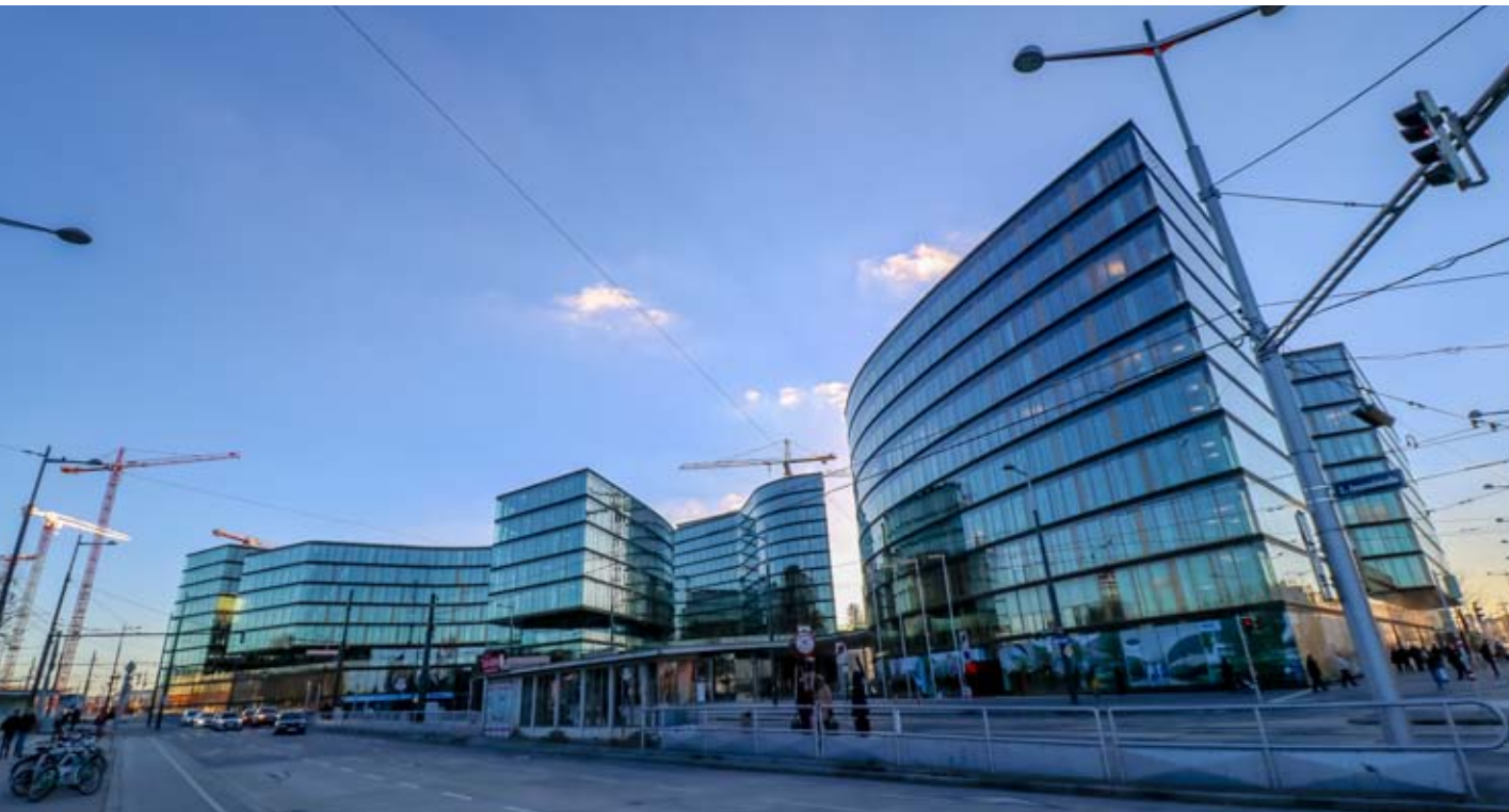
Vienna station, business offices
