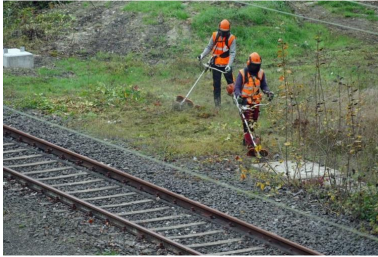
Figure 12: Lineside vegetation management using mechanical strimmers © Deutsche Bahn AG Volker Emersleben
