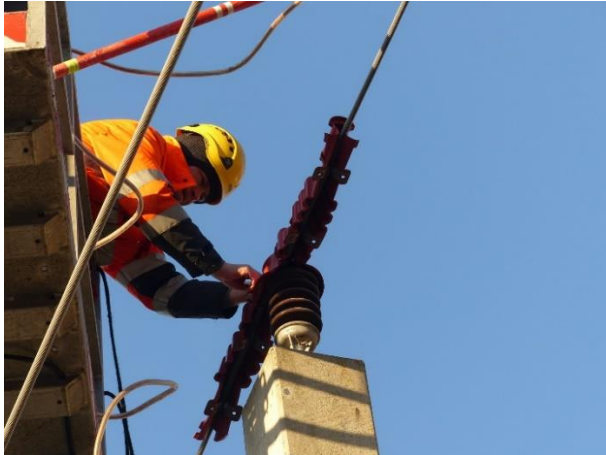
Figure 20: Bird protection caps on the overhead line masts © Renate Wunder, ÖBB-Infrastruktur, Austria
