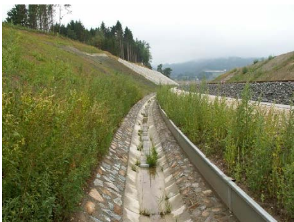
Figure 10: Trackside drainage ditch lined with concrete and stone.
