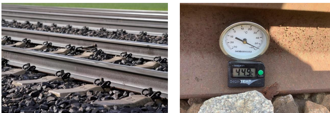
Figure 3: Left: A ballasted track with concrete sleepers. © Deutsche Bahn AG Daniel Saarboug, Right: A record-breaking forecast in the UK 53°C track temperature © Network Rail
