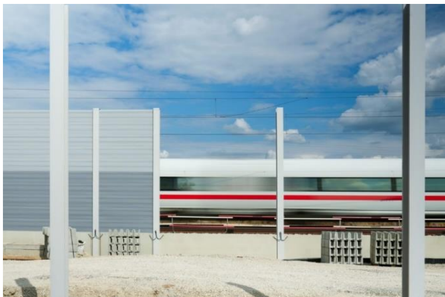
Figure 23: Installation of a noise barrier. © Deutsche Bahn AG Oliver Lang
