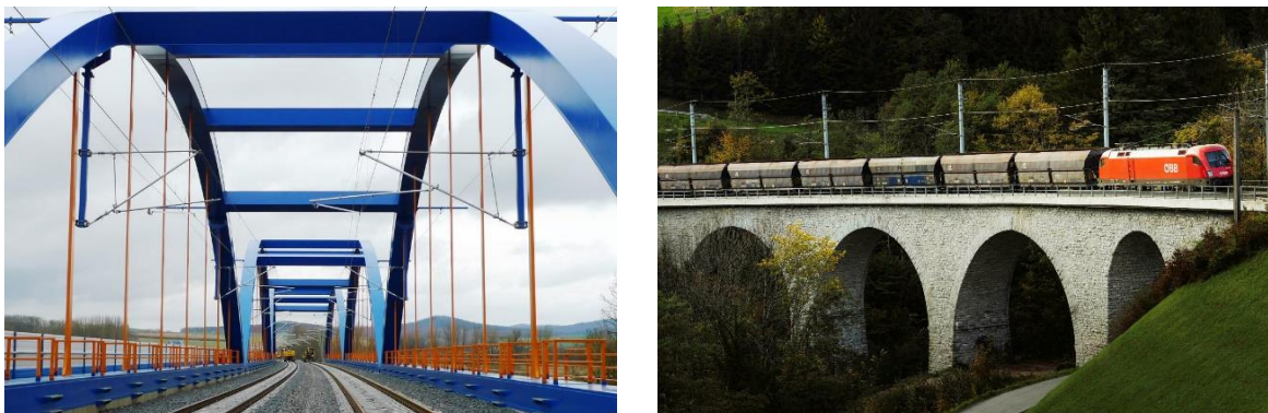
Figure 17: Bridge with closed construction. Left: © Deutsche Bahn AG Frank Kniestedt., Right: © ÖBB Rail Cargo, David Payr
