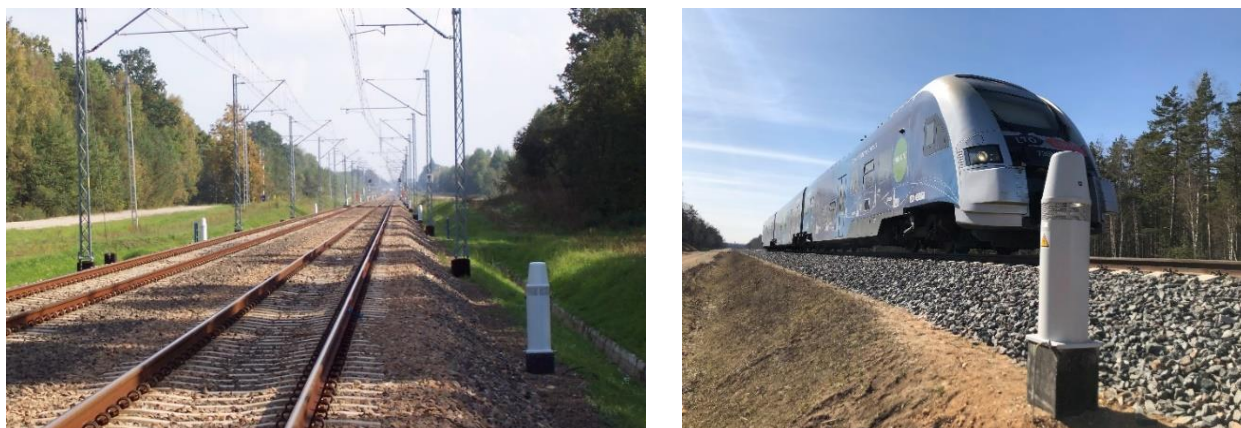
Figure 9: Animal deterrent system (left: E20 Line Warsaw, right: Lithuanian Railways), © NEEL, Poland
