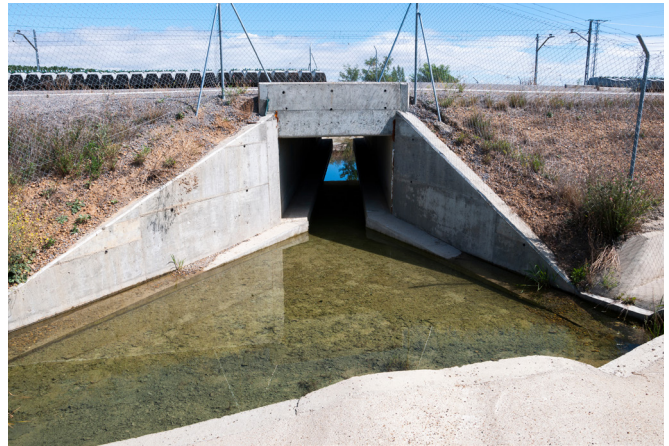
Figure 11: Examples of culverts that pass under the tracks and allow the passage of both water and animals © Jeff Ollerton & Adobe Stock
