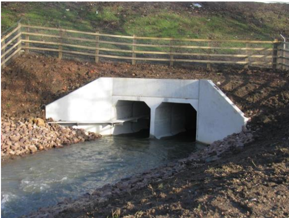
Figure 11: Examples of culverts that pass under the tracks and allow the passage of both water and animals © Jeff Ollerton & Adobe Stock
