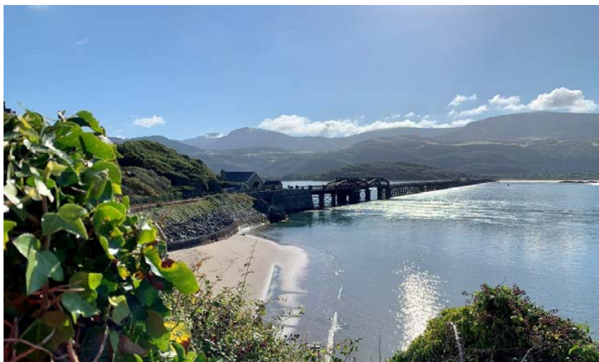
Figure 34: Coastal Area Railway and Bridge, © Network Rail
