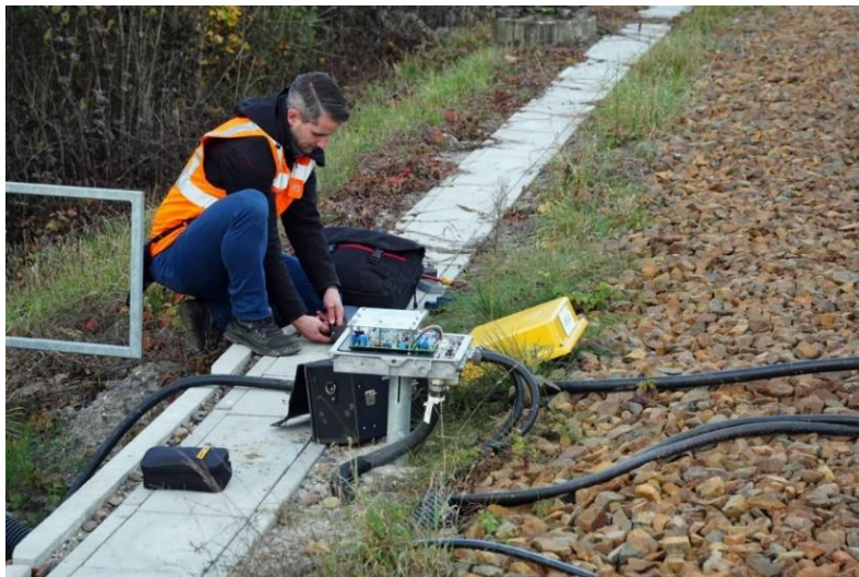
Figure 22: A closed cable channel. © Deutsche Bahn AG Volker Emersleben
