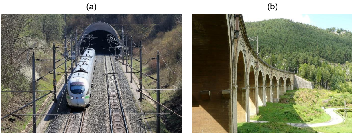
Figure 16: Example of a modern tunnel design as well as masonry arch viaduct a) © Deutsche Bahn AG / Wolfgang Klee, b) © ÖBB Infra AG
