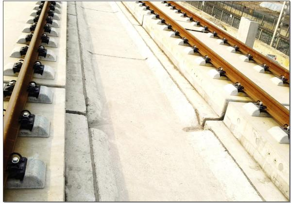
Aiming at over-limitation fastening gap at the end of the beam commonly seen in bridges with big spans in severely cold regions, proper design measures are adopted, as combined bedplate hanging at the bottom of the beam and setting abnormal track slab. Therefore, the problems can be solved.
