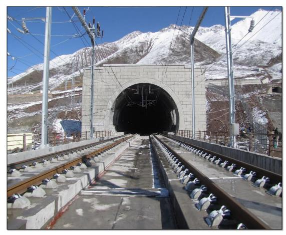
In the severely cold region, once the ballas tless track slab cracks, he ice-snow circula tion will expand the crack due to the freezi ng-thawing cycle. It will impair the service I ife of track slab Therefore, the CRTSI ball astless track slab structure is developed, w hich adopts the biaxial prestressed track sl ab to avoid the occurrence of cracks on the track slab's surface, by doing this, unfavor able influence of frost heave on the track st ructure can be effectively reduced.
