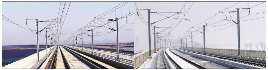
In design, it takes full consideration of frost resistance of reinforced concrete base. In the subgrade, bridge and other open-line sections, transverse expansion joints are set every 1 to 2 rail slab of the base, which forms a unit structure. Standard of filling material between the expansion joints in ballastless track structure is developed.
