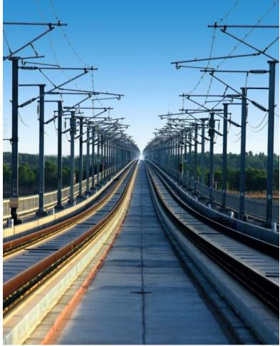
Taking into account the frost resistance, rail platform is provided at the fastener fulcrum position to reduce the snow and ice impact on the fastener system. The adoption of 'composite board' structure, made of self-compacting concrete and track slab, improves the durability of the track structure.
