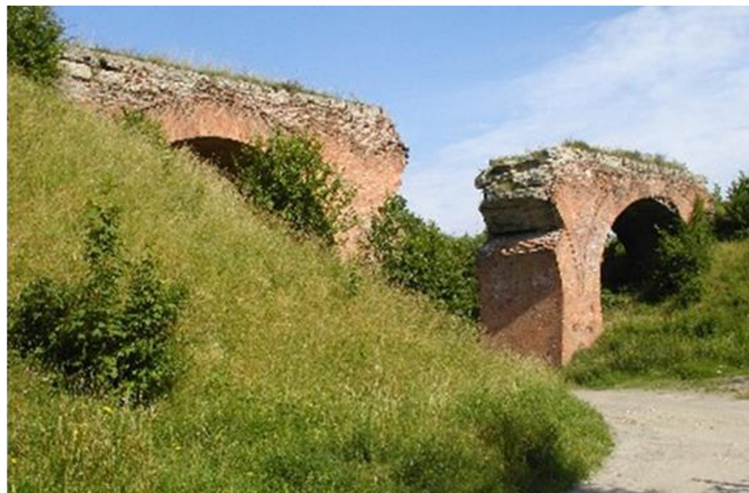
A viaduct in Gdansk Bretowo, 2004
