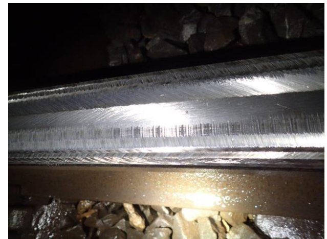
Rail after acoustic grinding
