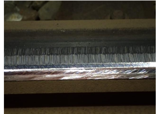
Rail after regular grinding
