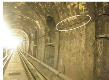
Photo 10 - Area of missing and eroded string course to Down side wall at south end.
