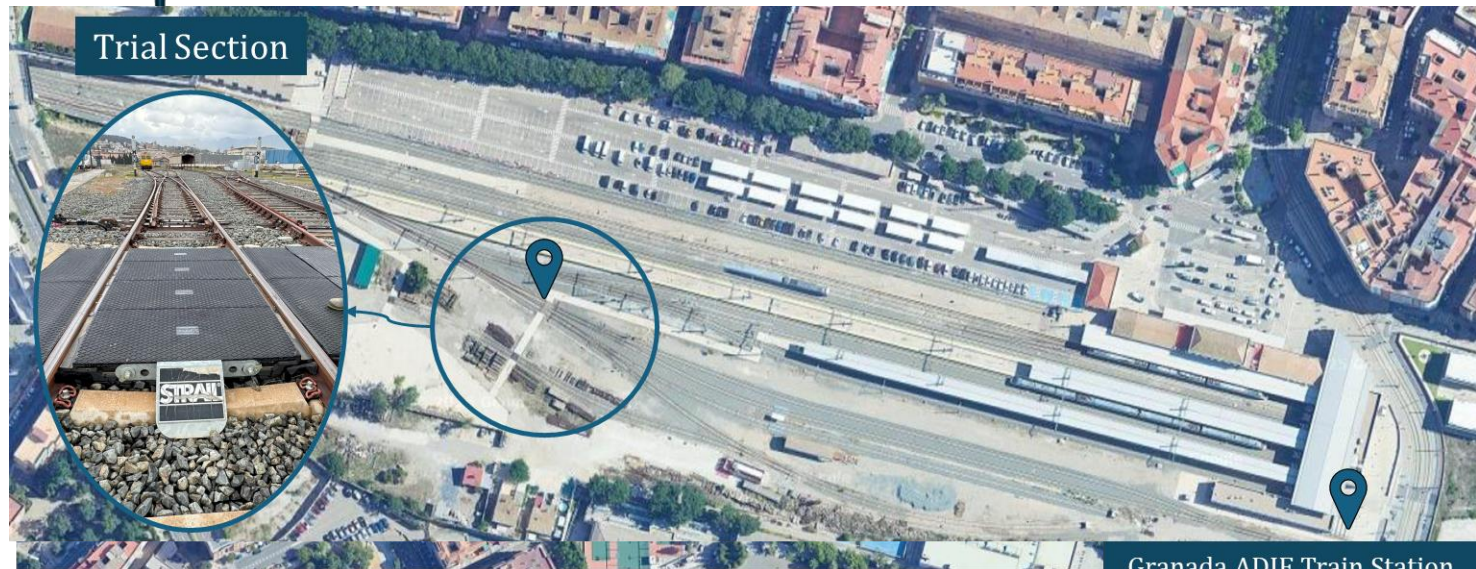
Granada ADIF Train Station
