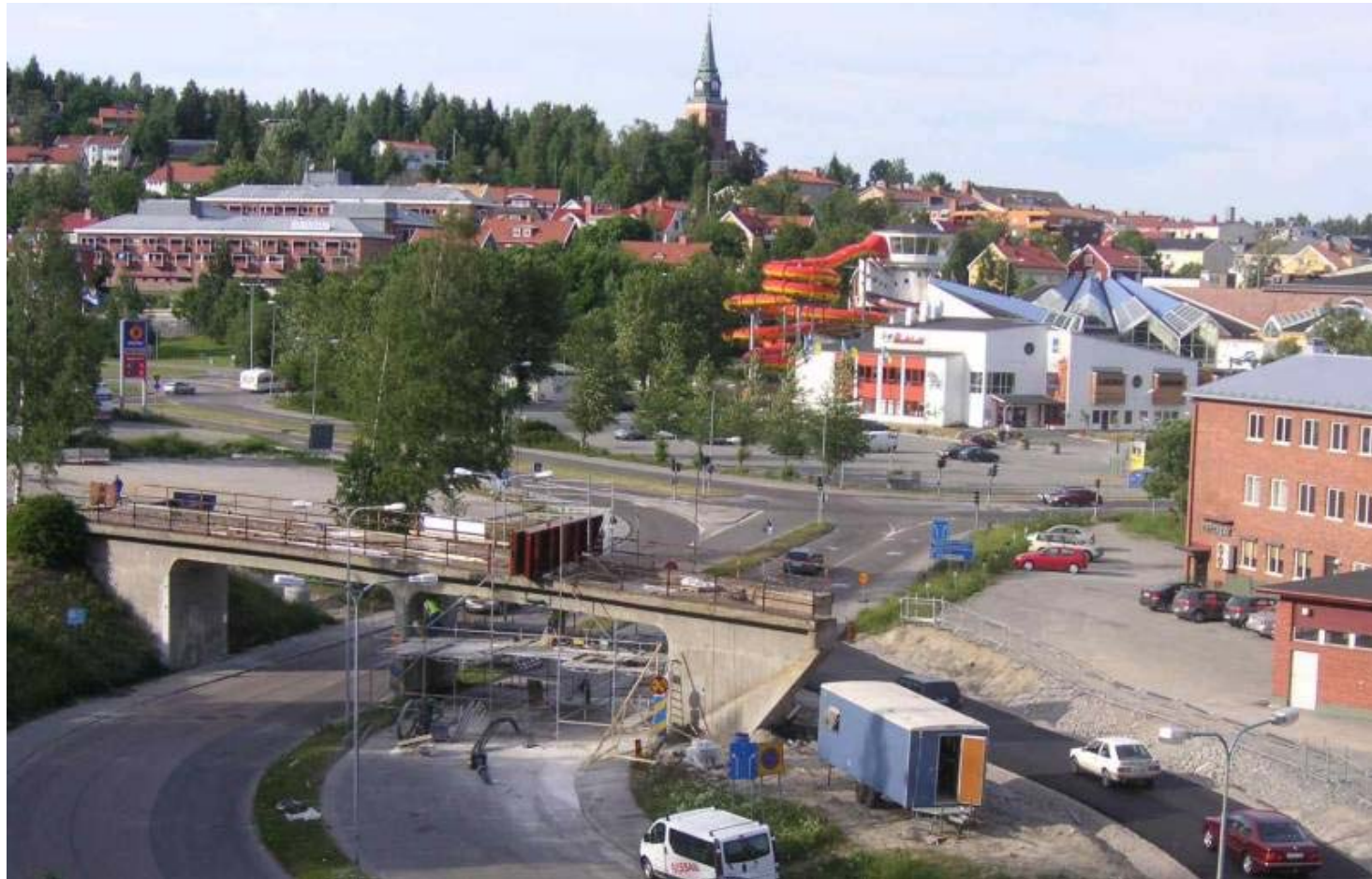
Testing of a strengthened R C Bridge 2006 in Örnsköldsvik, Sweden
