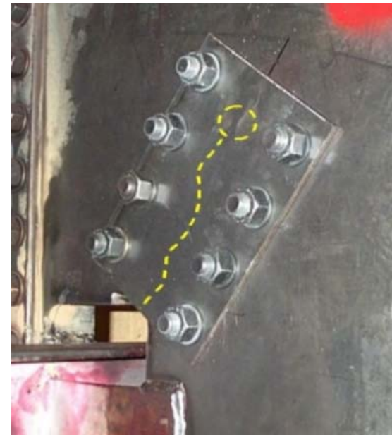
Bolted steel doubler
